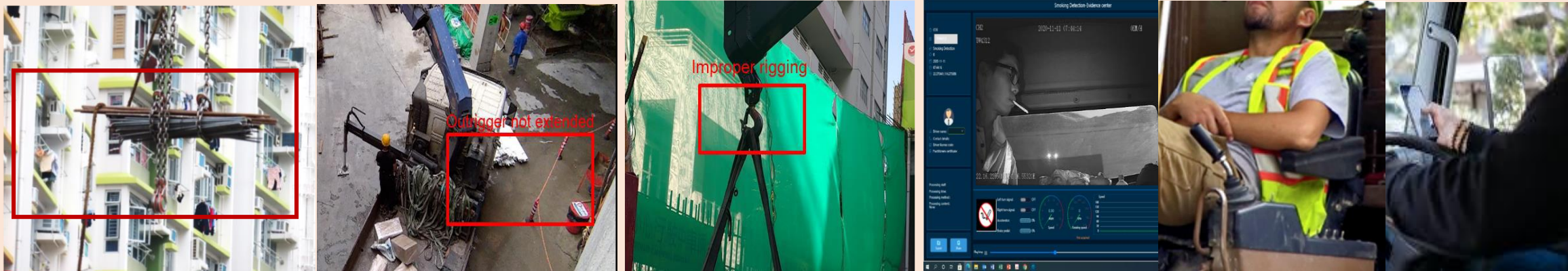
Detecting proper application of lifting method, outrigger and lifting gear, inappropriate behaviour of operator by AI
